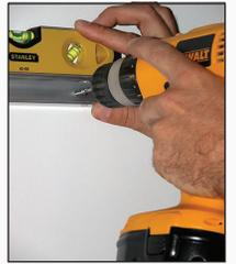
Place the frame on the C-rail and line up the proper holes in the frame with the holes in the C-rail and slide the clevis pins in place.
