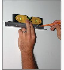
Using a 5/32nd drill bit, drill holes at the marked locations or just screw self tapping drywall anchors into the wall where the pencil marks are.
